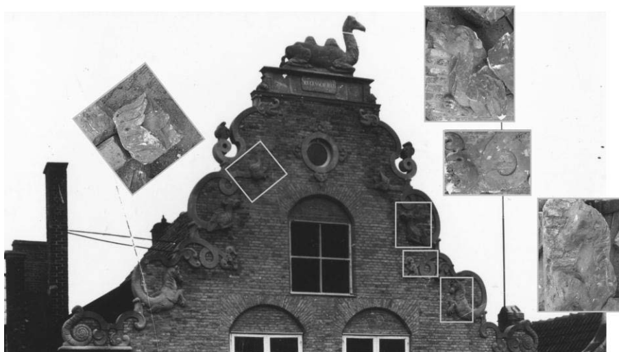
Fig. 3. Front gable elevation of the Camel House; pre-1945 state [source: Registry of the Department of Urban Planning and Architecture in Elbląg]. Original decorative elements found on 06.03.2022 during archaeological surveys
